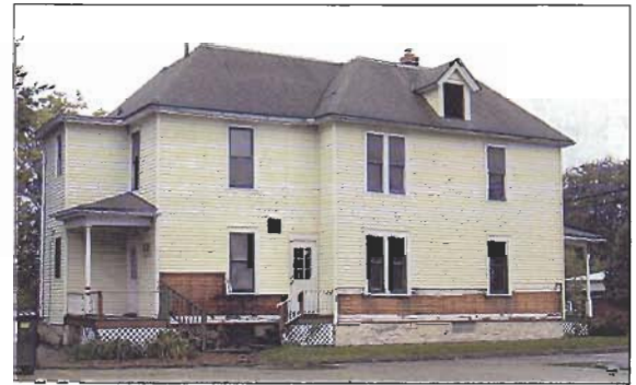
Photo (2): Side of home preparing for demolition.
